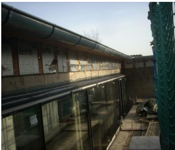
Figure 5: Office window of outbuilding
